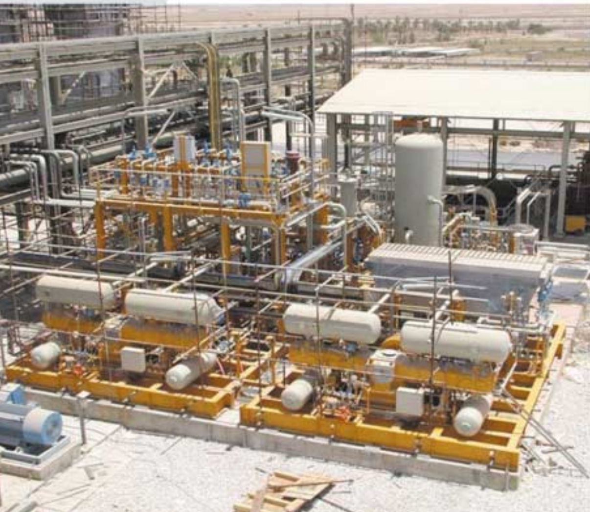
FUEL GAS BOOSTING UNIT BUILT ACCORDING API 618 LOCATED IN MIDDLE EAST
